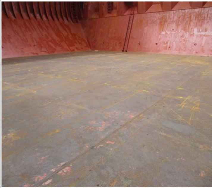
1. Hold Nr. 3 tank top plating was found clean and dry.
