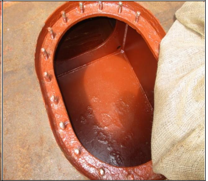
4. Hold Nr. 3, bilge well Ps, found clean and dry.
