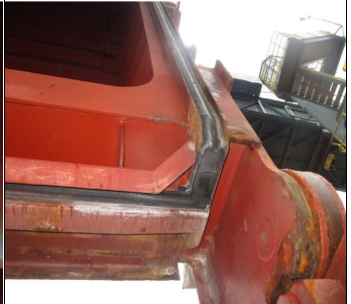
10. Hatchcover in hold Nr. 3, rubber packing in good conditions.
