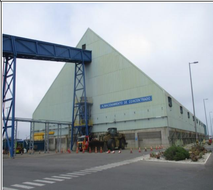
11. View of stockpile.
