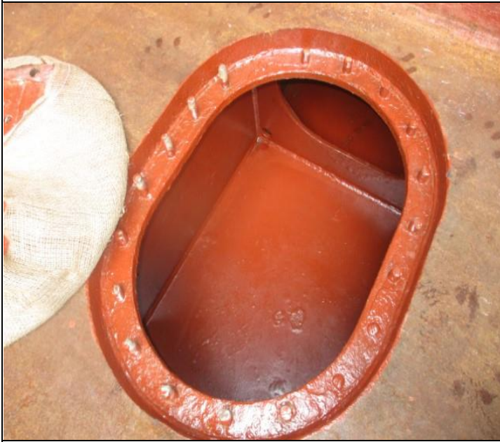
3. Hold Nr. 3, bilge well Ss found clean and dry.
