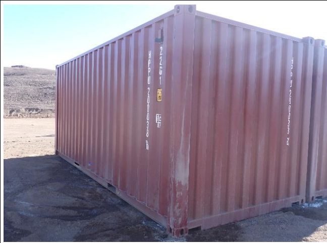
5. Side panel in good conditions.
