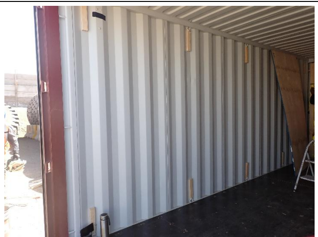
12. Wooden used in the lined.
