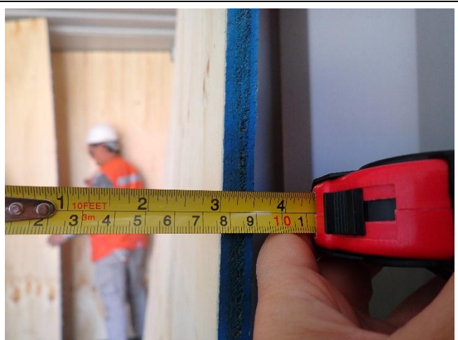
16. Measure of wood 12 mm.
