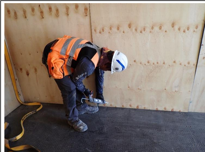
15. Silicone to isolate nails.
