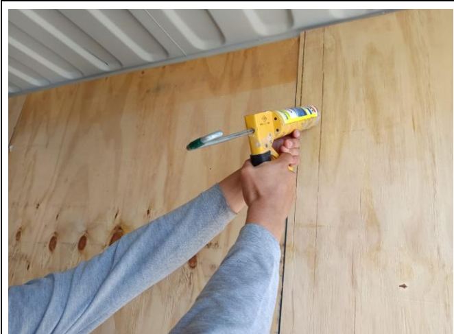
15. Silicone to isolate nails.
