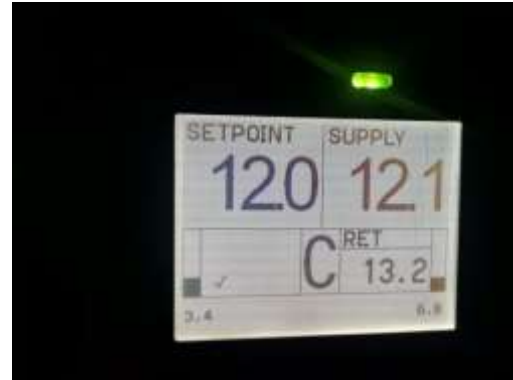
22. Set point and return temperature at the time that the stuffing finished.
