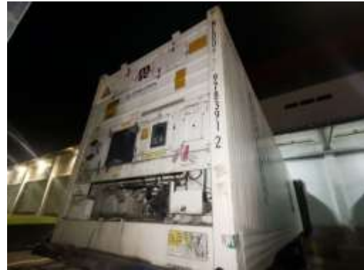
6. Fan housing on the refrigerated container.
