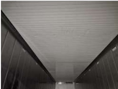
11. Ceiling of the container.
