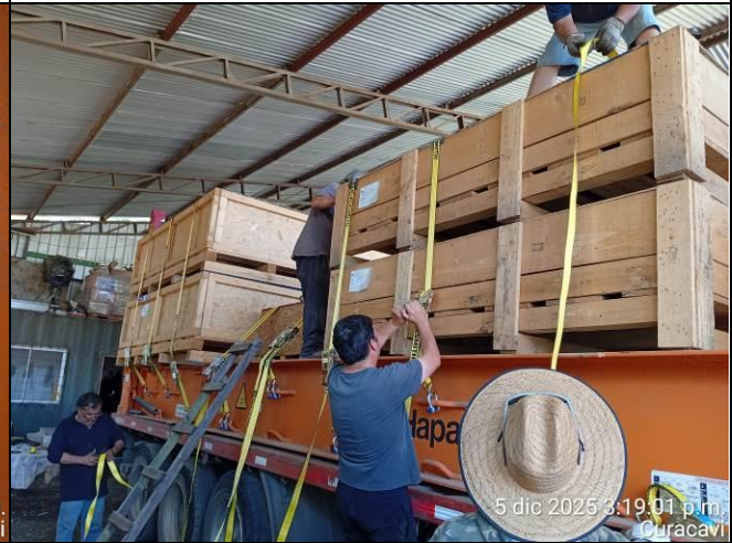
4. View of lashing operations with slings.
