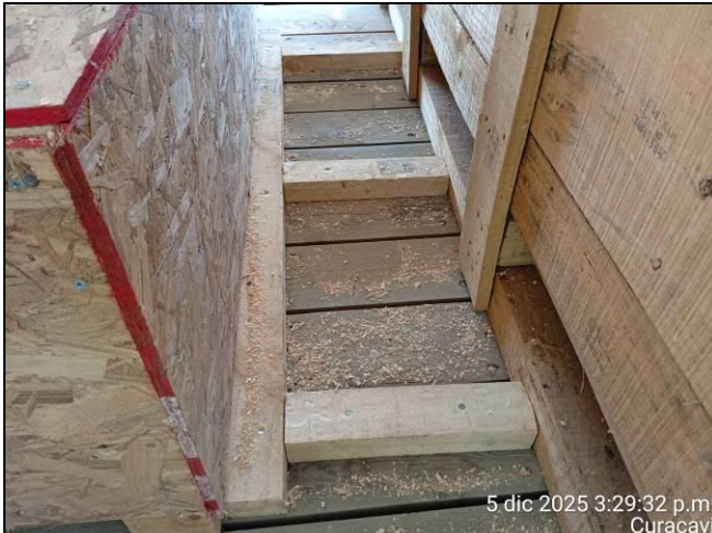
9. Crates were chocked by means square ladders.
