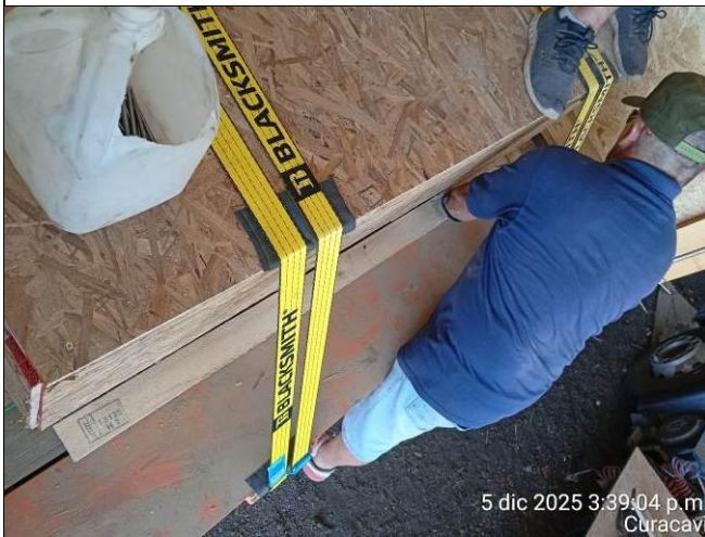
3. Square lumbers for chocking being installed.
