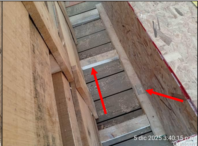
10. Square ladders used for chocking duly stamped.
