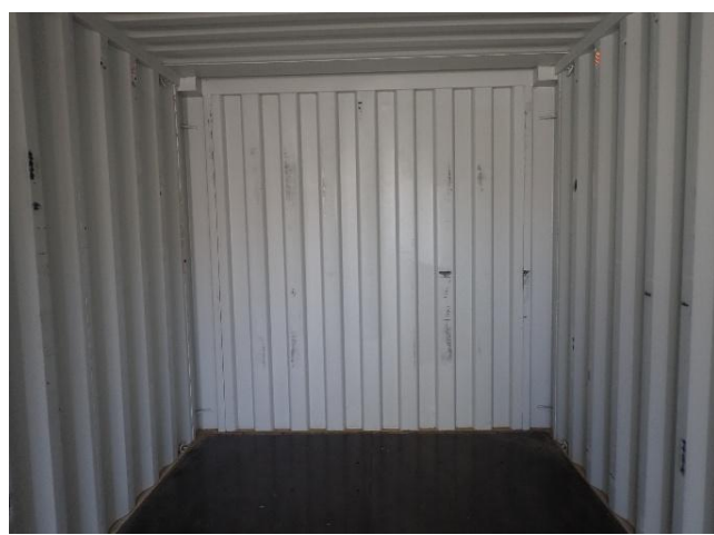
7. Container floor in good conditions.
