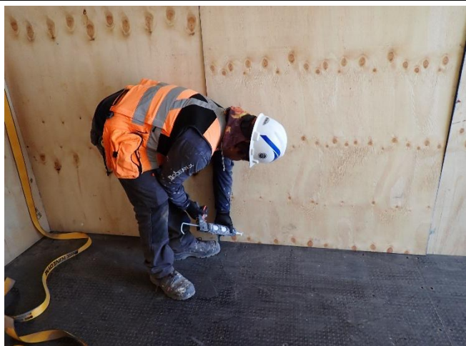
15. Silicone to isolate nails.
