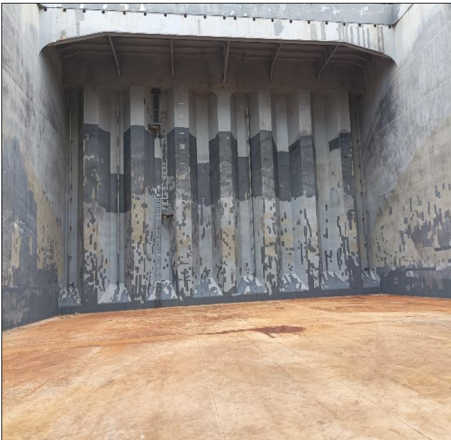
2. Hold Nr. 2, general condition of bulkhead/Fwd.
