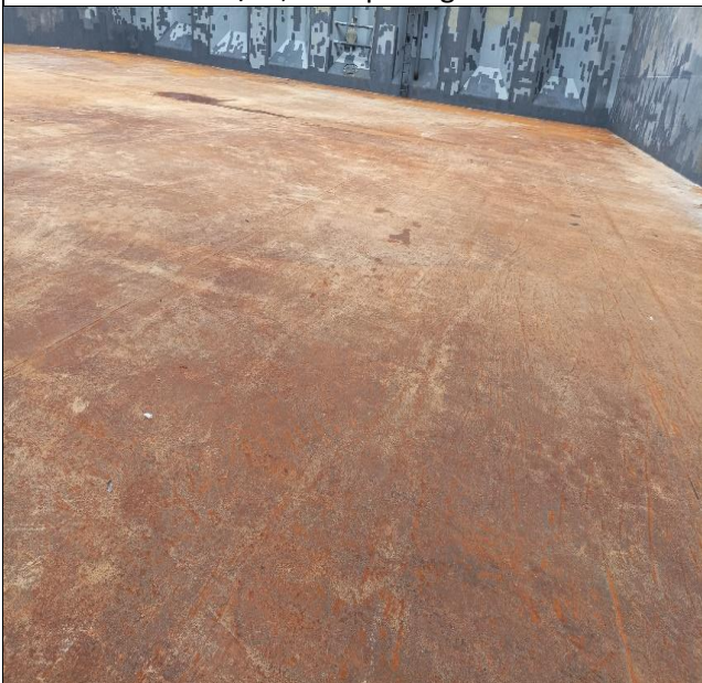
6. Hold Nr. 2, general condition of tank top plating.
