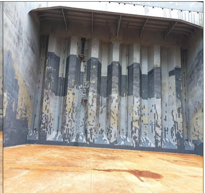
3. Hold Nr. 2, general condition of bulkhead/Aft.
