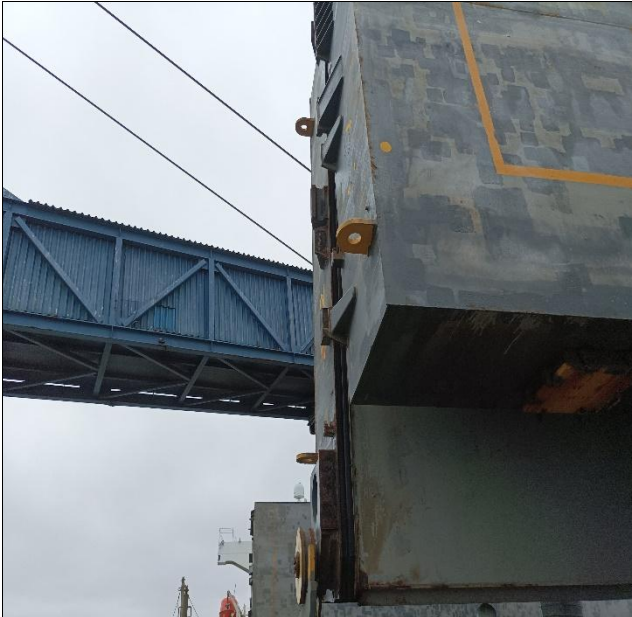
20. Ship loader system located in hold Nr. 2.
