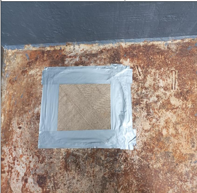
10. Hold Nr. 2, bilge/Ss covered with burlap and sealed with tape.
