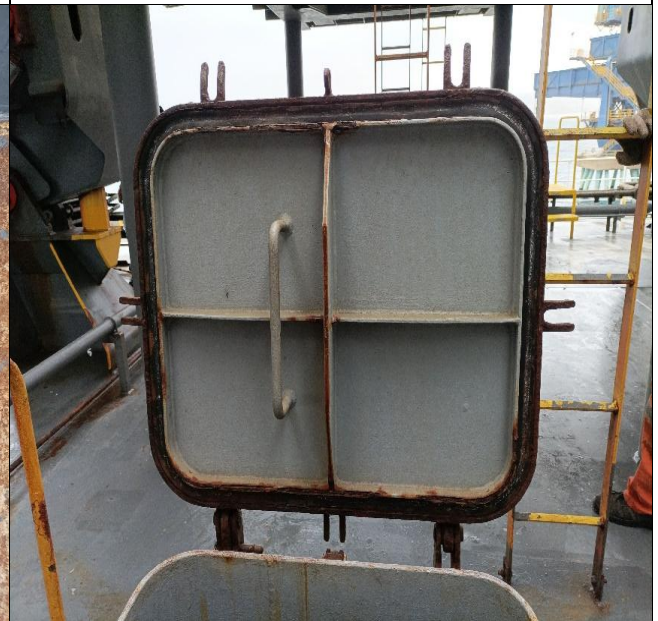
11. Hold Nr. 2, stevedores' access with rubber packing in good conditions.
