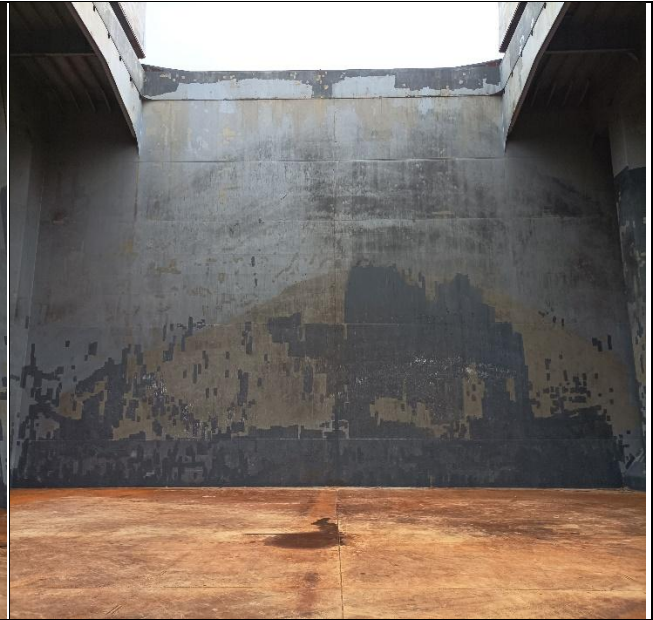
5. Hold Nr. 2/Ss, shell plating condition.
