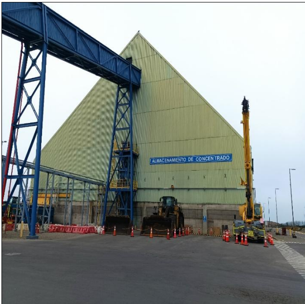
18. View of stockpile warehouse.
