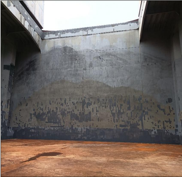
4. Hold Nr. 2/Ps, shell plating condition.
