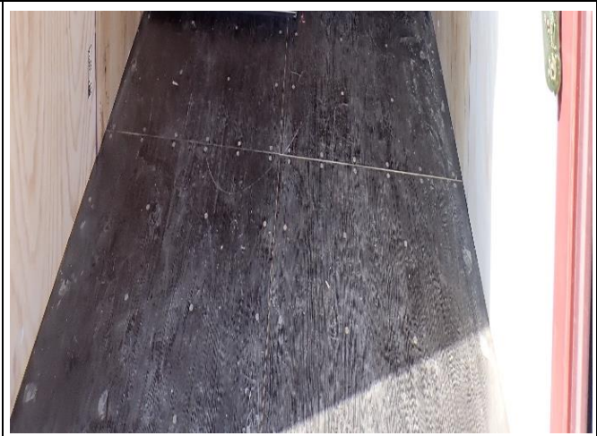
6. Container floor in good condition.
