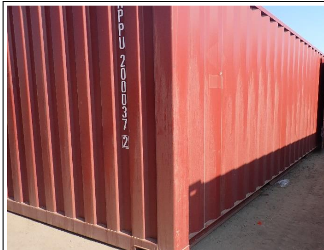
3. Side panel in good condition.
