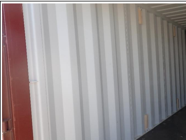
7. Roof panel in good condition.
