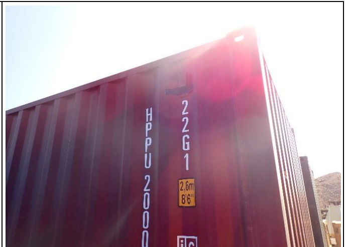
4. Corner fitting and frontal panel in good condition.
