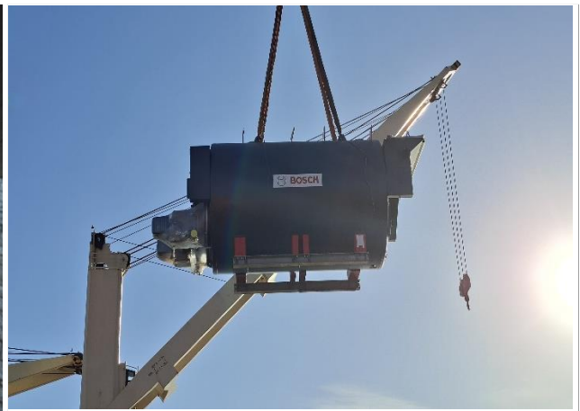
14. Boiler being discharged from the vessel
