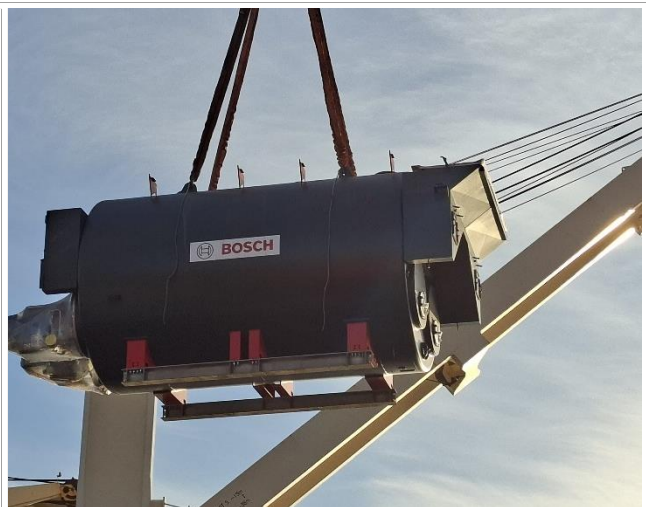
20. Boiler in the process of being discharged from the vessel
