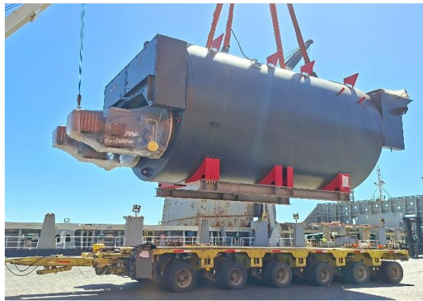
9. Boiler being discharged alongside the vessel.
