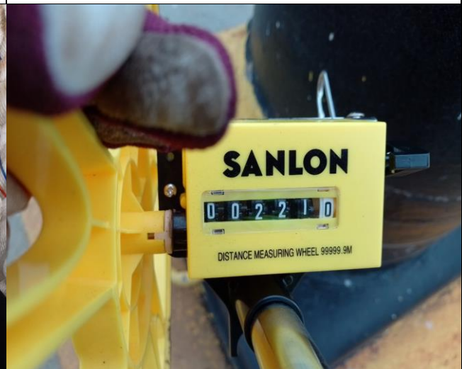
44. Length measured by surveyor.
