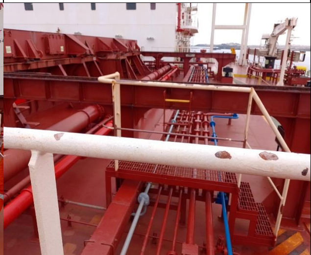
44. View of spring Btw 8-9 Pedestal Roller Guide.
