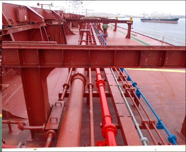
48. View of spring Btw 3-2 Pedestal Roller Guide.
