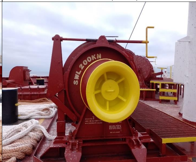
8. View of winch for brest line.
