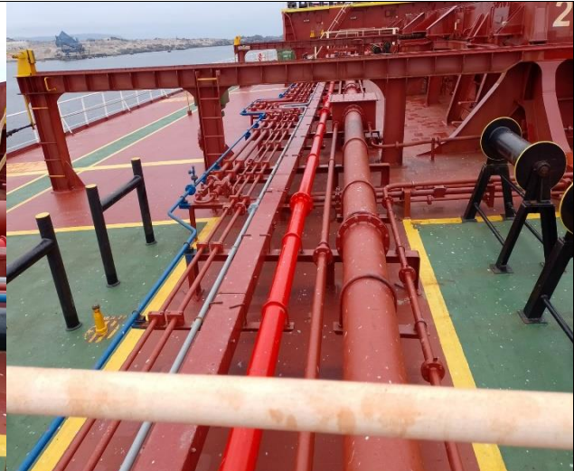
46. View of spring Btw 3-2 Pedestal Roller Guide.
