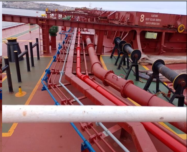
42. View of spring Btw 8-9 Pedestal Roller Guide.
