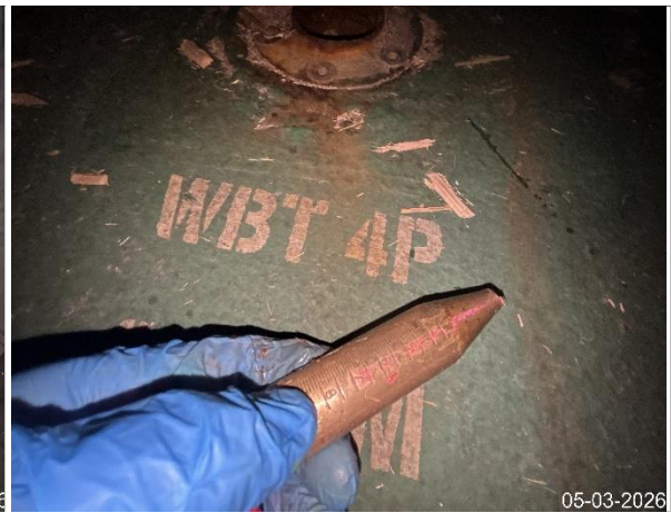
22. Continue checking the ballast.
