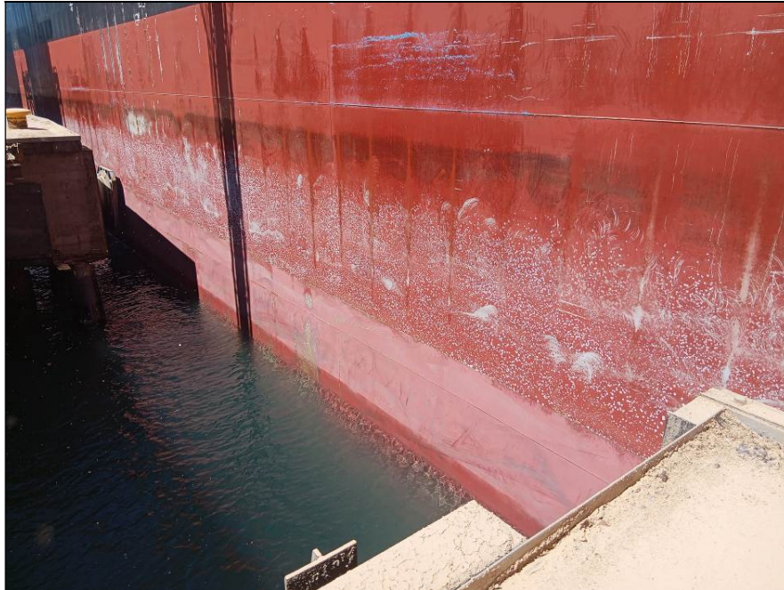
5. Hull, Mid. section; paint scratched and rusty.
