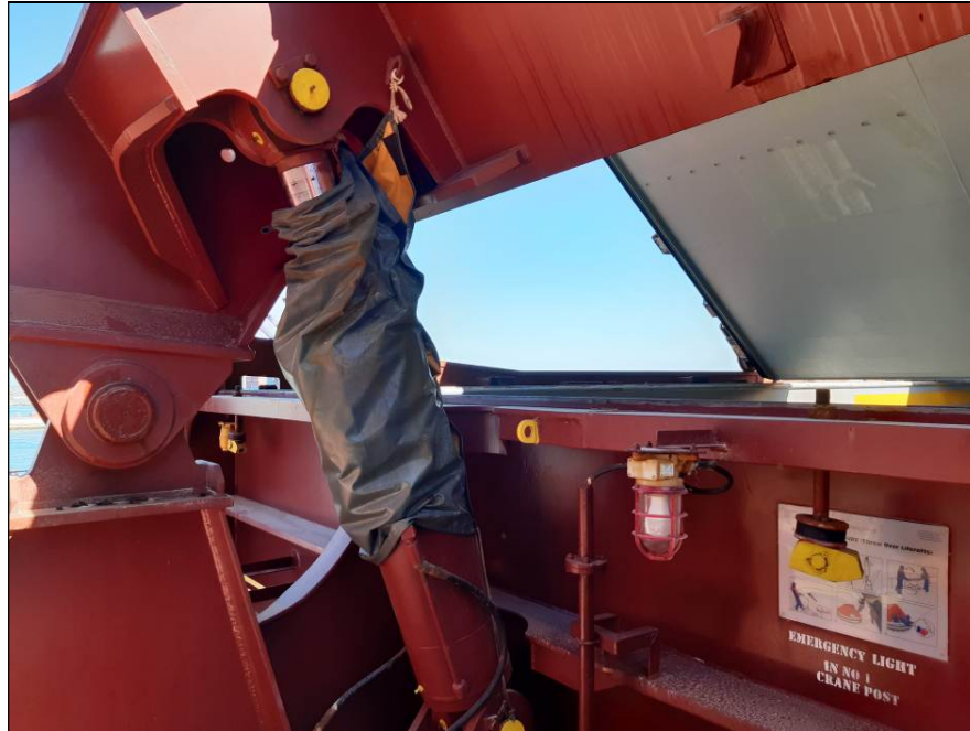
35. Hatchcover No. 1, hydraulic systems in good conditions
