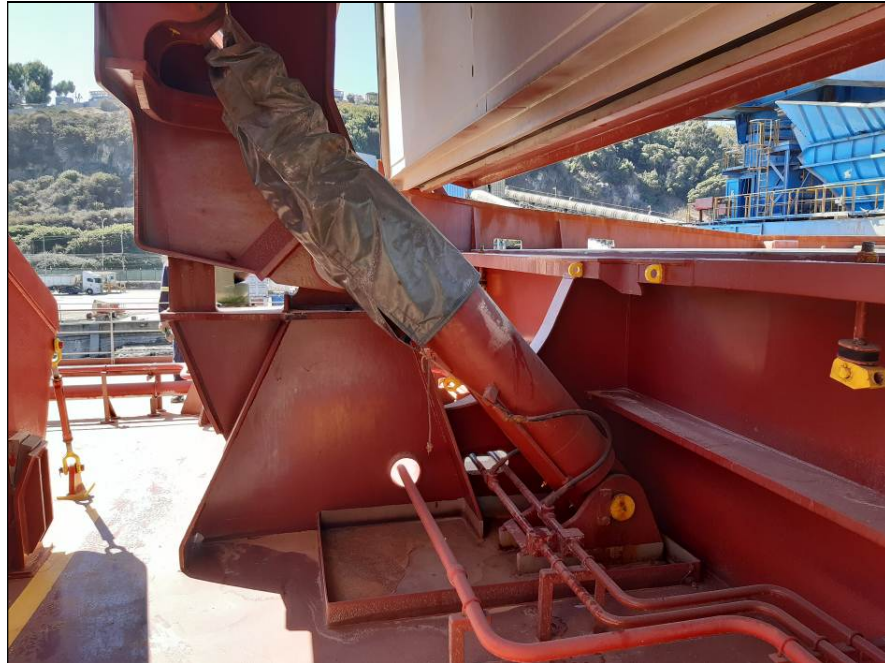
43. Hatchcover No. 2, hydraulic system in good conditions.
