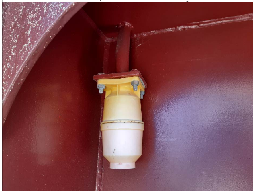
62. Hatchcover No. 4, non-return valves in good conditions.
