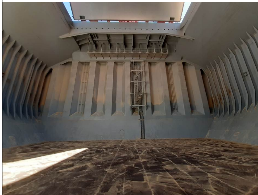
66. Fwd bulkhead with paint scratched.
