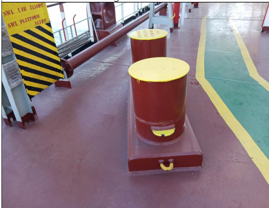
26. Bollards in good conditions.
