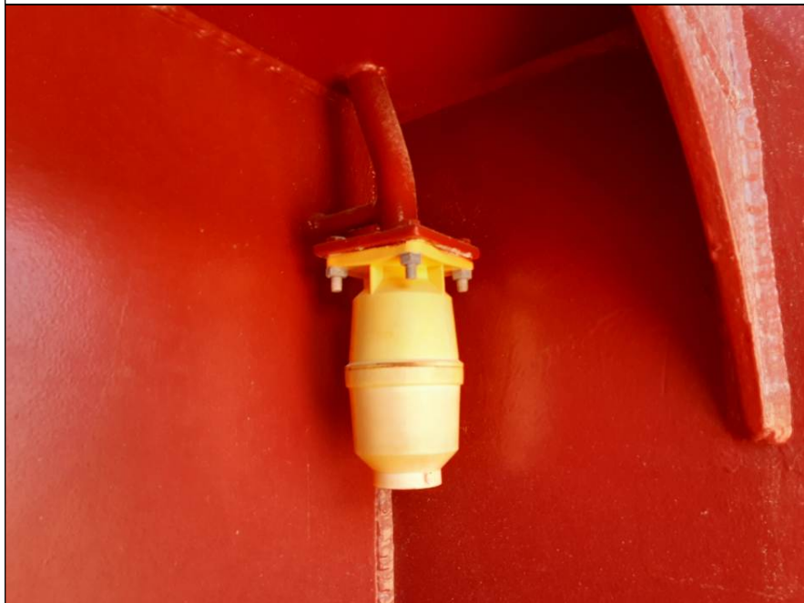
40. Hatchcover No. 2, non-return valves in good conditions.
