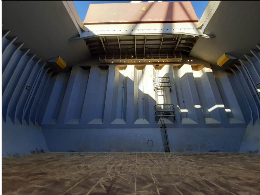
57. Aft bulkhead with paint scratched.
