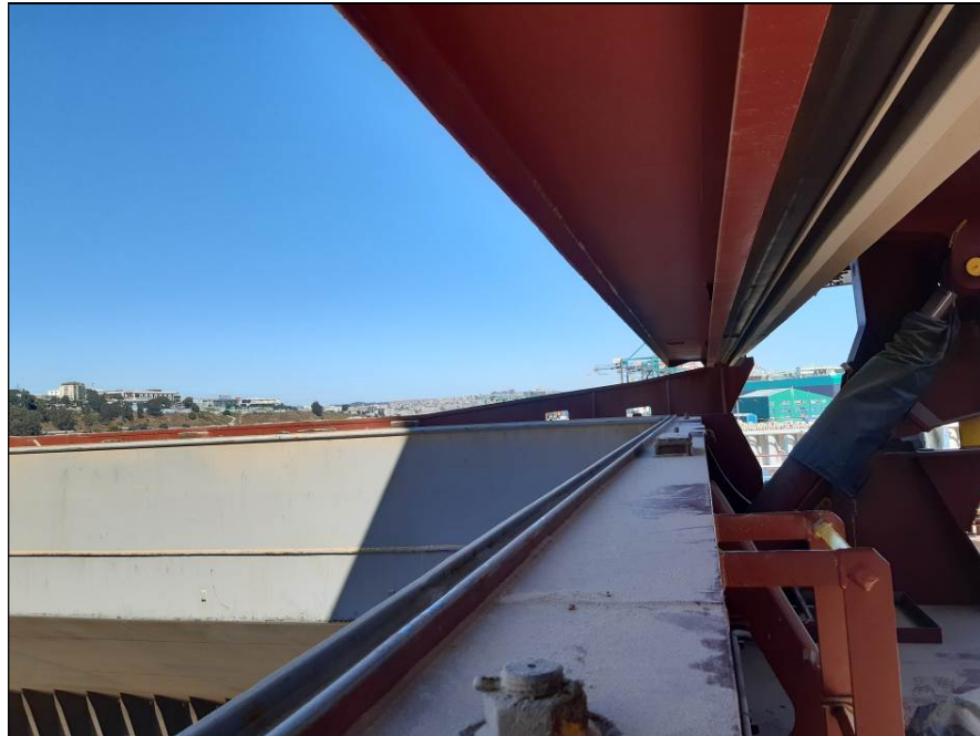
63. Hatchcover No. 4, rubber gasket in good conditions.
