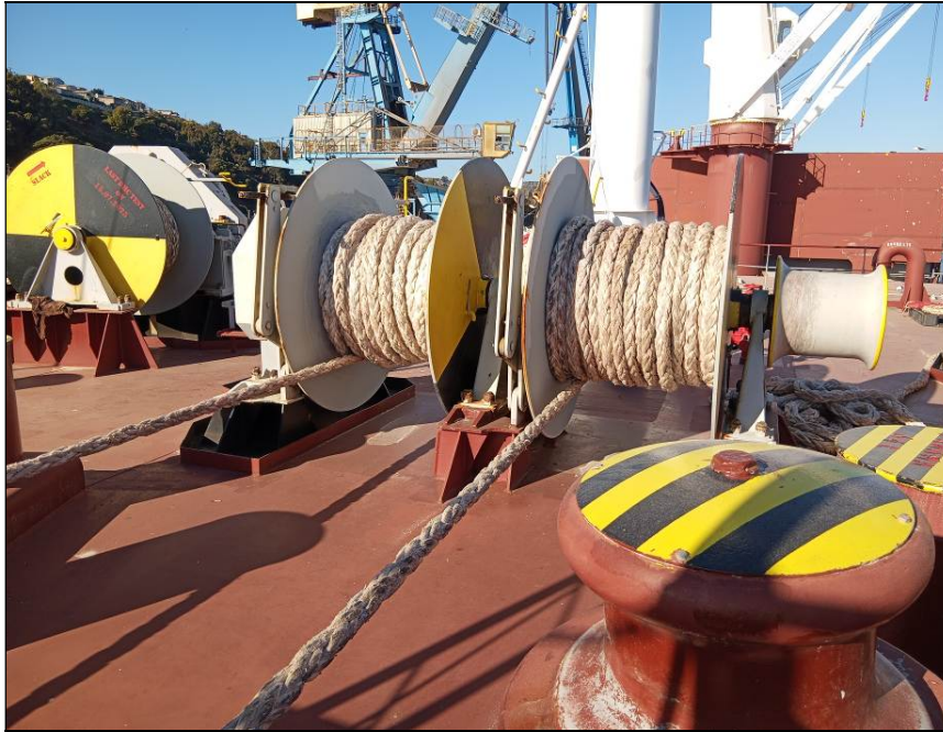
19. Center winch, in good conditions.
