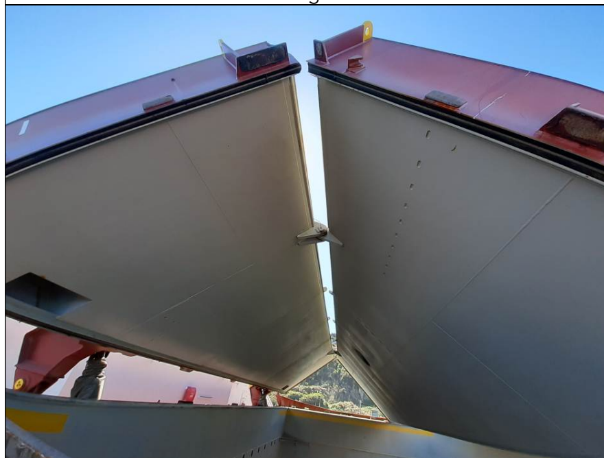
34. Hatchcover No.1, rubber gasket in good conditions.
