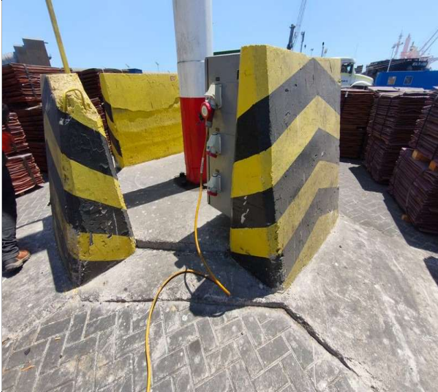
21. Container RF HC HLBU 617420-0 connected to terminal power supply.
