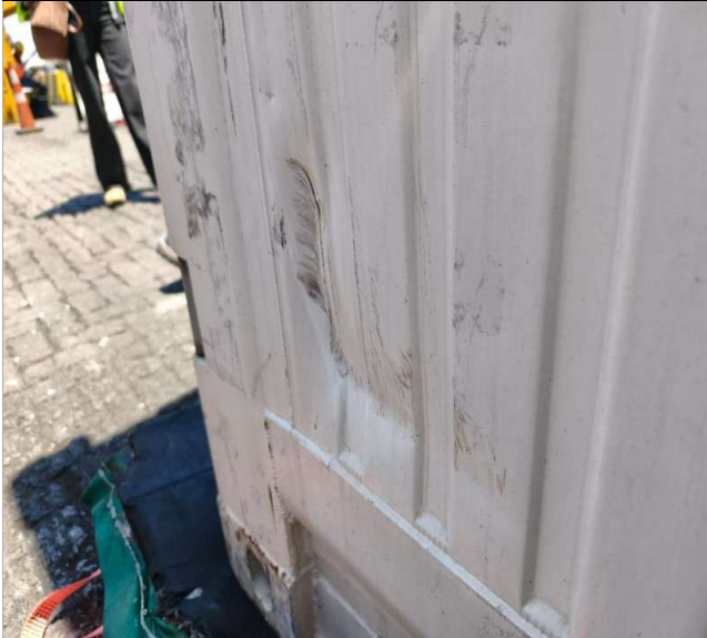
13. 1x40' RF HC HLBU 617420-0 right panel with scratches and dented. Section 0 lower part
