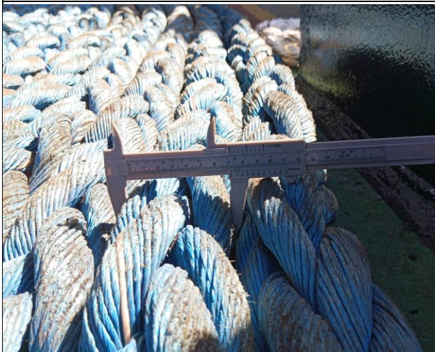
11. View of diameter measurement of the mooring lines.
