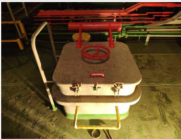
12. - View of seal in hold N°4 (AFT)
