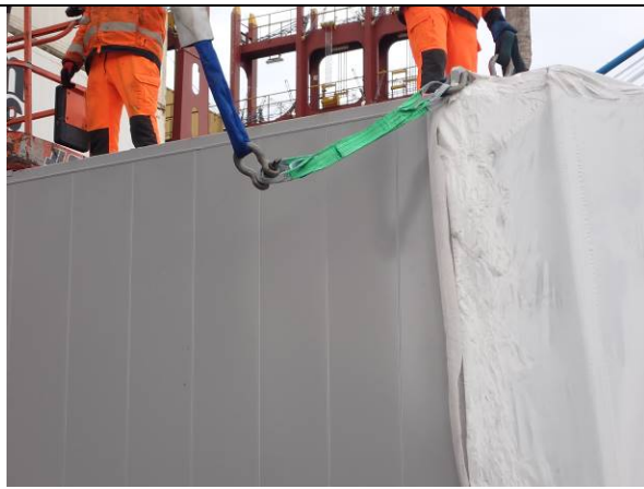
Lifting with rigging modified and correct
