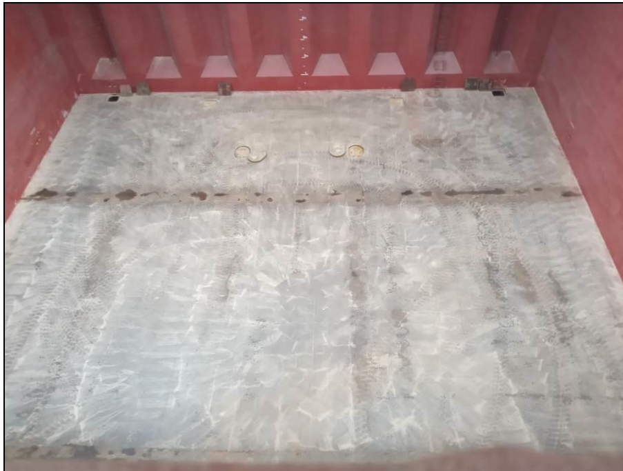
47. General view of C/H N° 3.
