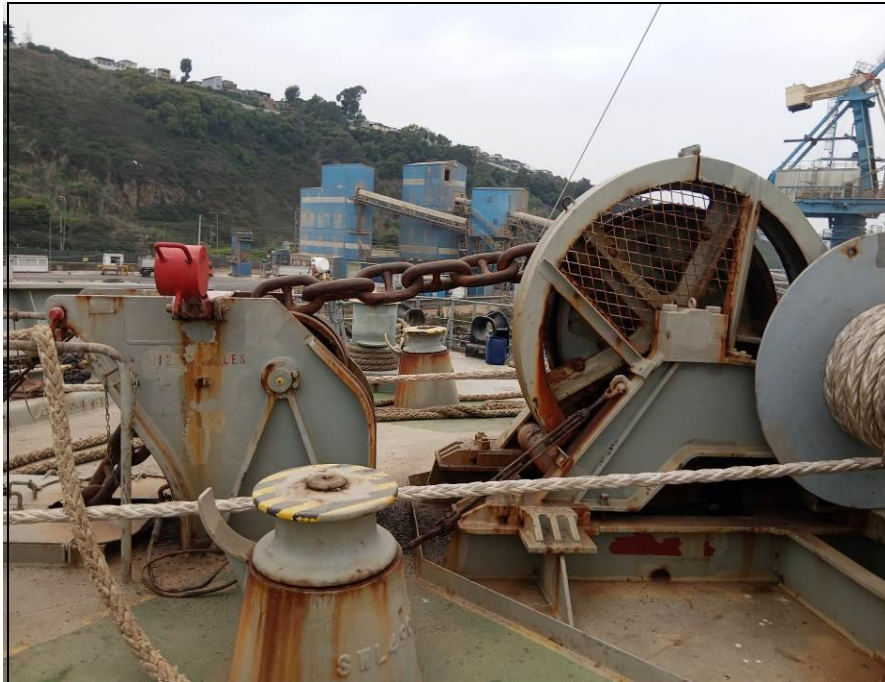
19. Ss capstans, in good conditions.
