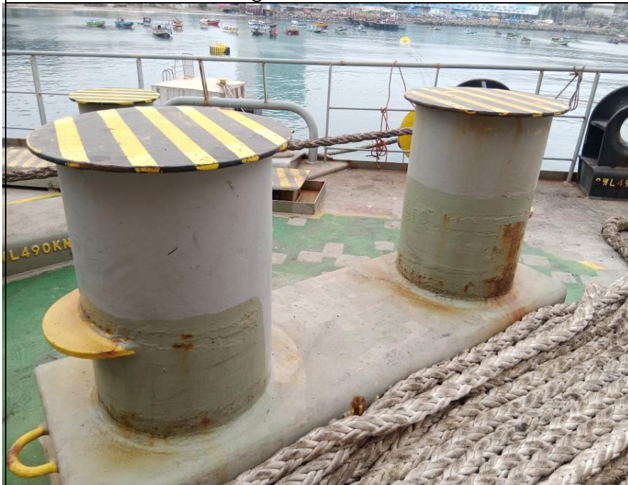
26. Bollards in good conditions.
