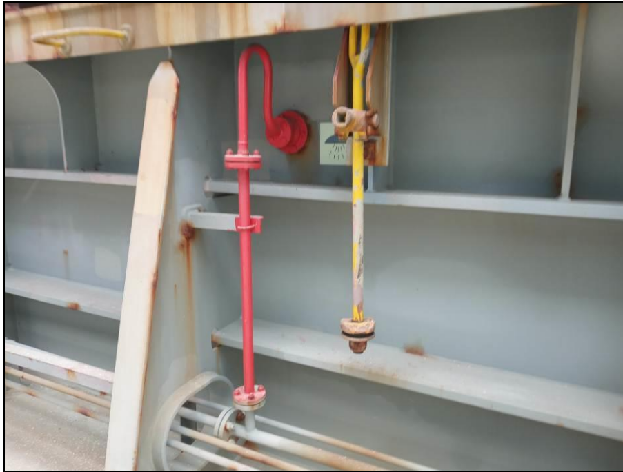
55. Hatchcover No. 3, active cleat in good conditions.
