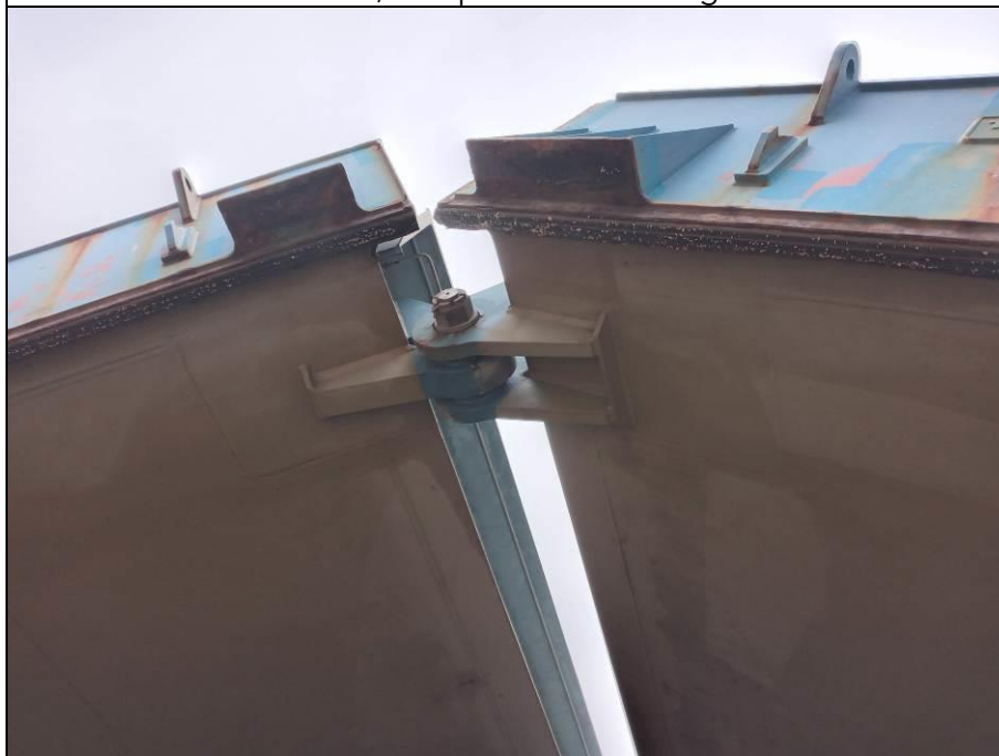
76. Hatchcover No. 5, rubber gasket in good conditions.
