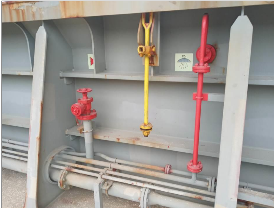
63. Hatchcover No. 4, active cleats valves in good conditions.
