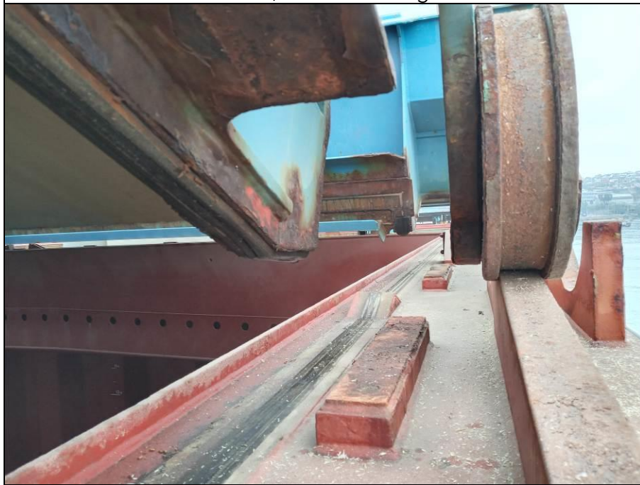
56. Hatchcover No. 3, compression bars in good conditions.
