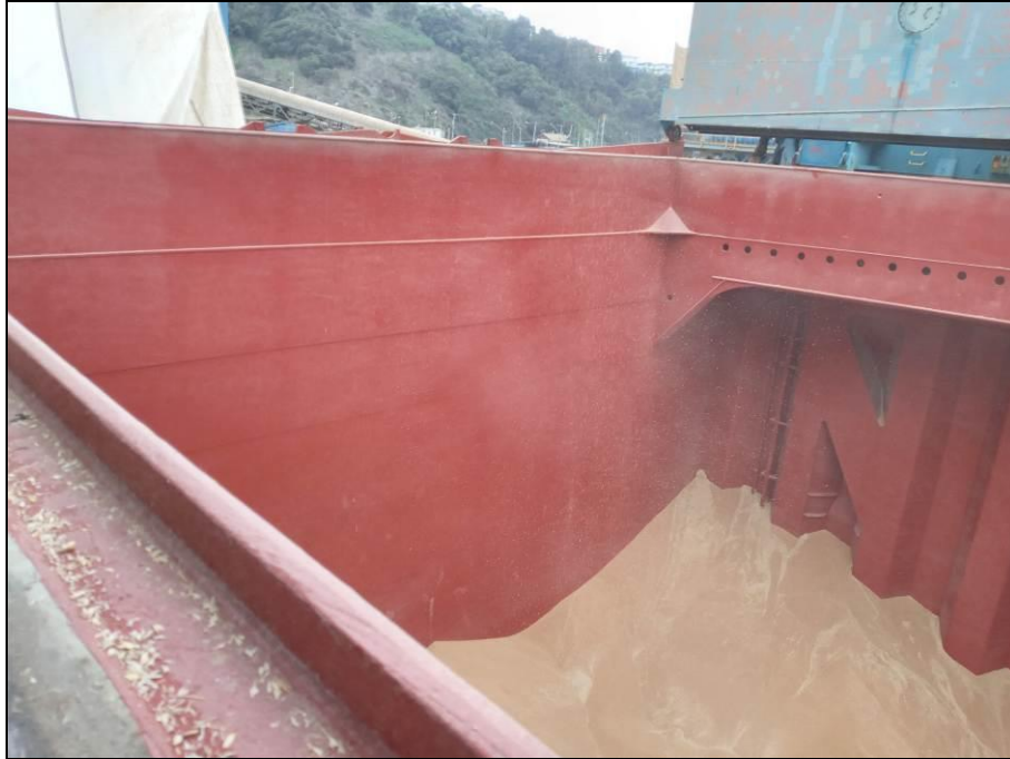
61. Side/shell plating Ss, with paint scratched and rust.
