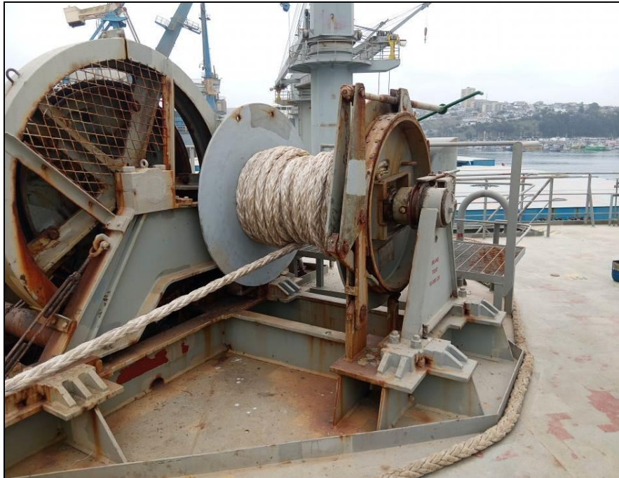
15. Winch Ss Fore deck, in good conditions.
