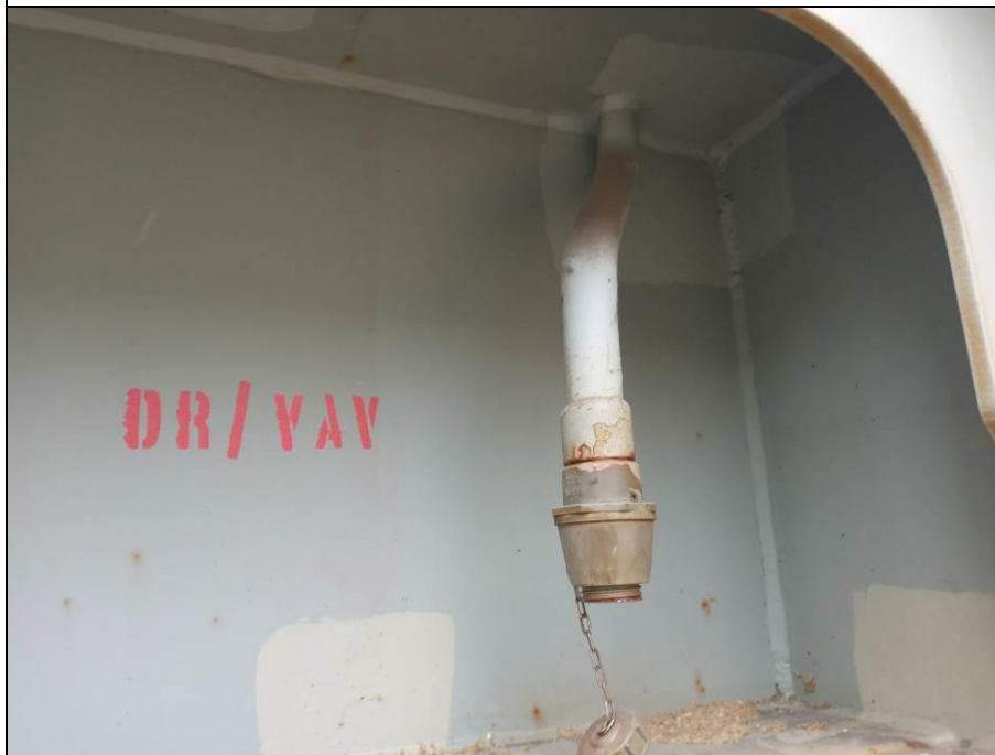
44. Hatchcover No. 2, non-return valves in good conditions.
