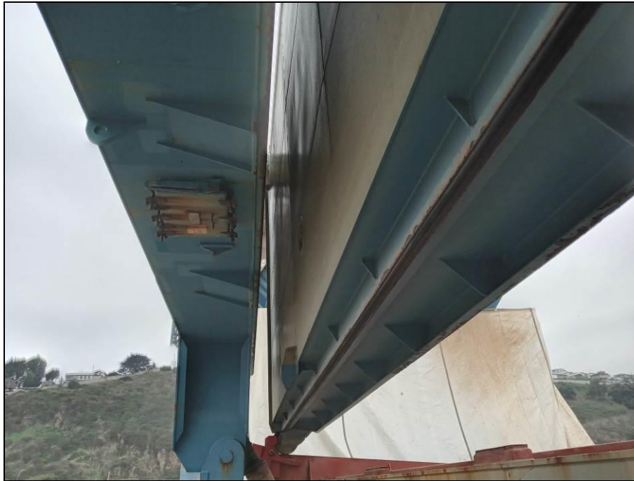
65. Hatchcover No. 4, rubber gasket in good conditions.
