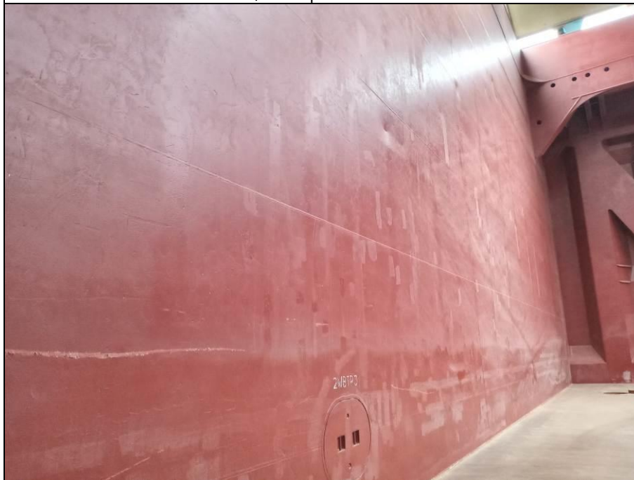
40. Side/shell plating Ps, with paint scratched and dust.
