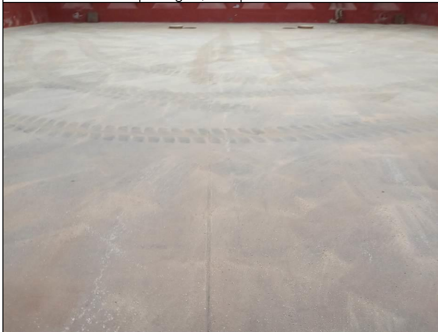
42. Tank top plating with dust.
