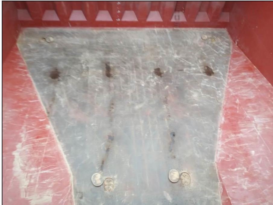
67. General view of C/H N° 5.
