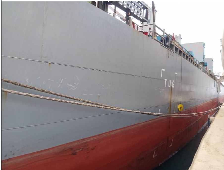
12. Aft to fwd view.
