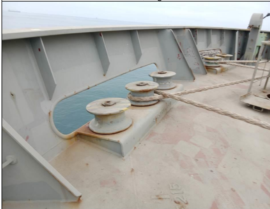
16. Roller guides in good conditions.
