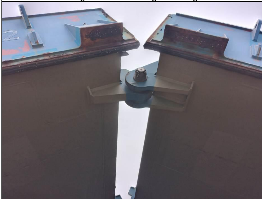
34. Hatchcover No.1, rubber gasket in good conditions.
