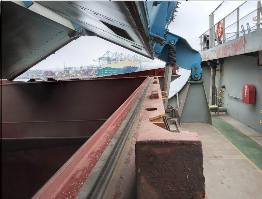
36. Hatchcover No. 1, compression bars in good conditions.
