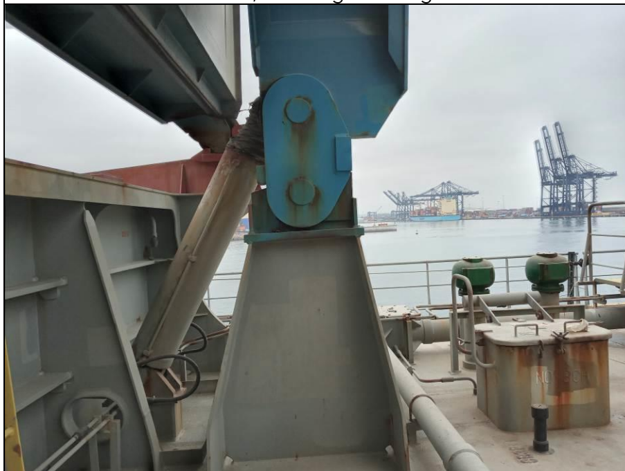
66. Hatchcover No. 4, hydraulic system in good condition conditions.
