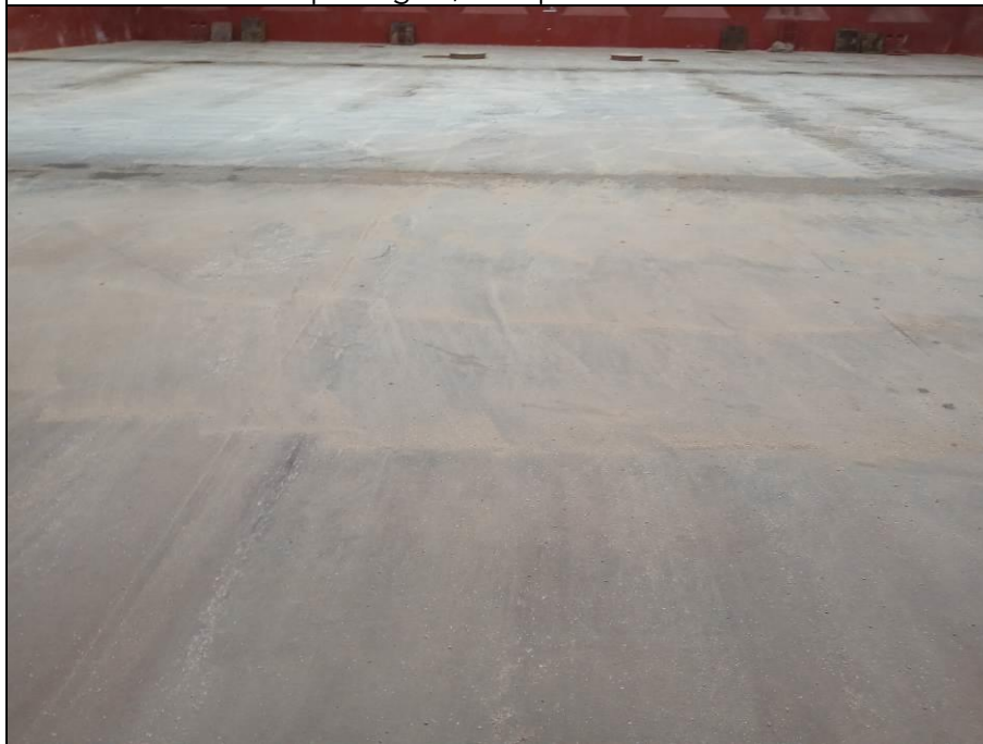
52. Tank top plating with dust.
