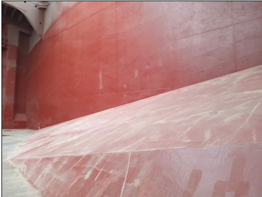
71. Side/shell plating Ss, with paint scratched and rust.
