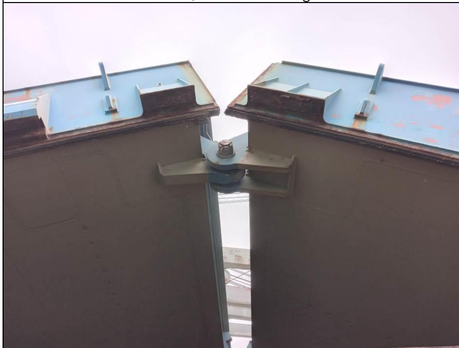
46. Hatchcover No. 2, rubber gasket in good condition.
