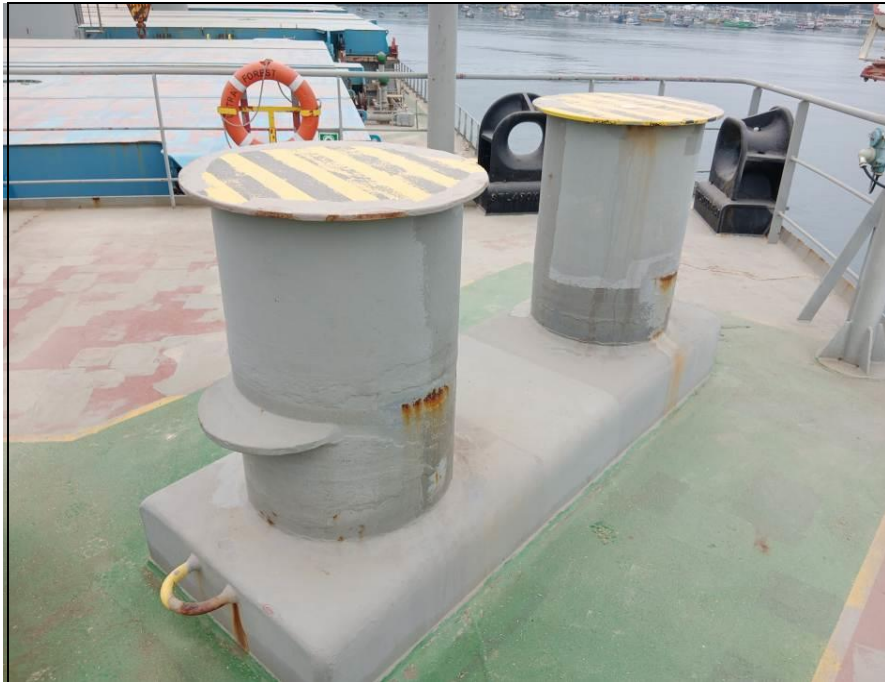
17. Bollards in good condition.
