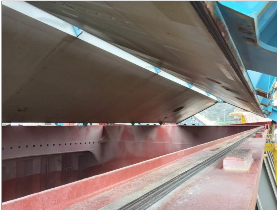
75. Hatchcover No. 5, compression bars in good conditions.
