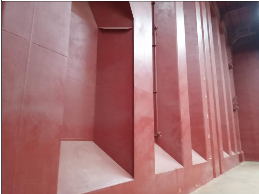
38. Fwd bulkhead, with paint scratched and dust.
