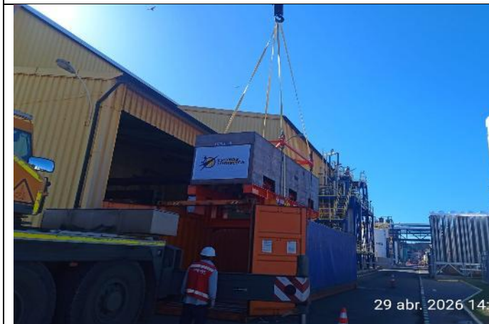
3. View of stuffed electrolyzer into OT container
