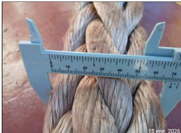
5. View of diameter measurement of the mooring lines.
