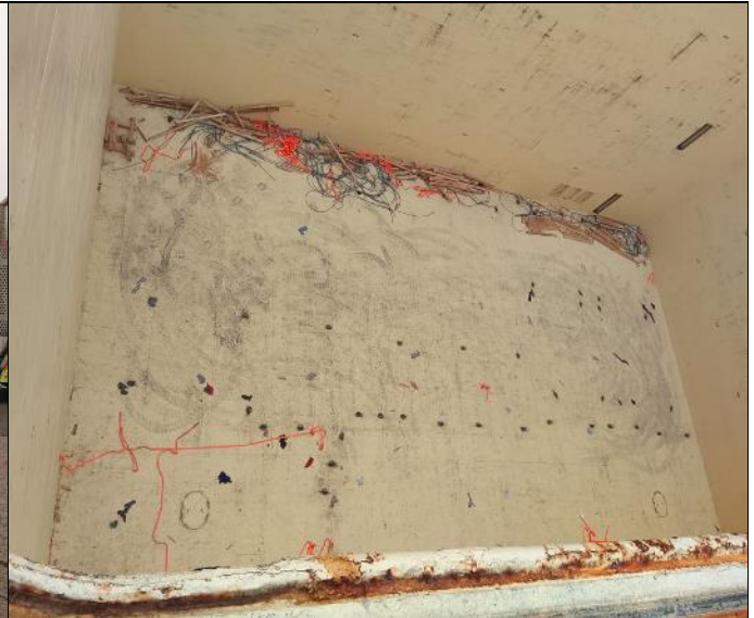
58. Bodega No. 5 rematada.
