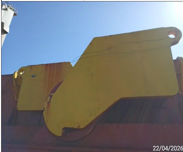
3. Hold Nr. 2, general view of hatch cover sealed.
