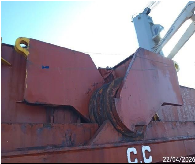
9. Hold Nr. 4, general view of hatch covers sealed.
