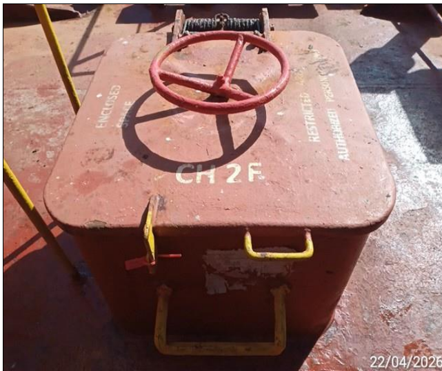
1. Hold Nr. 2, general view of stevedore's access, Fwd sealed.
